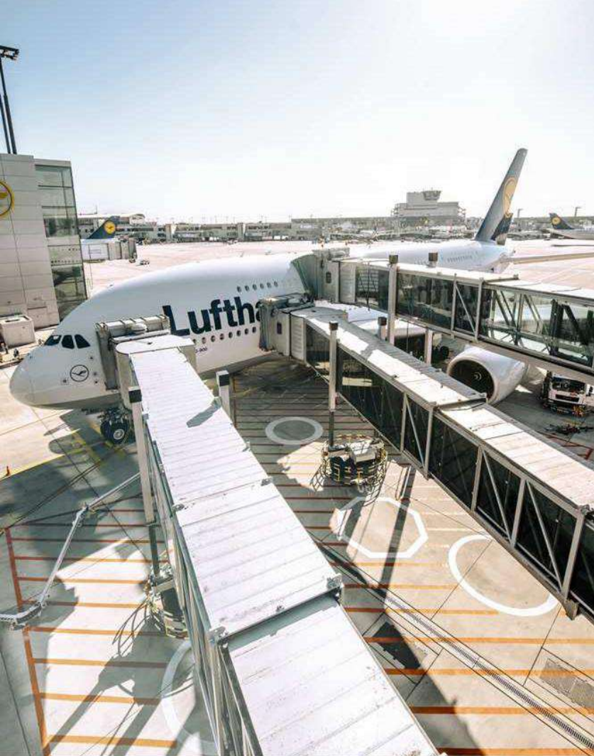
PASSENGER BOARDING BRIDGES
